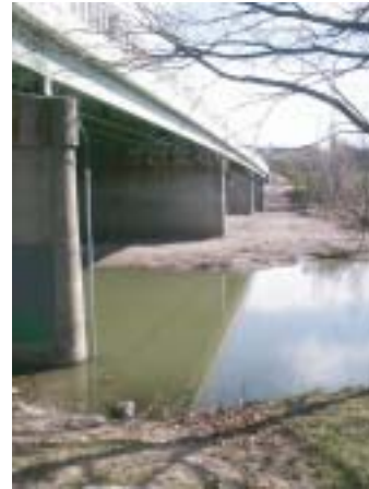
Highway bridge, downstream face
