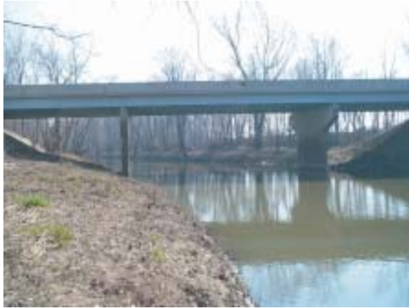
View, looking upstream
